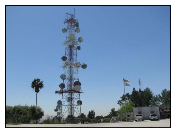
Figure-7: Co-location of equipment by Service Providers
